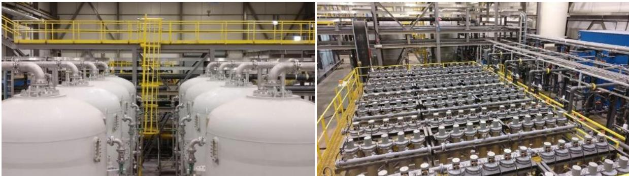
**Figure 2: IX and ERC Circuits – Kemess Selen-IX™ Plant**
