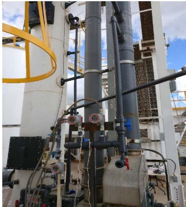
Figure 3. Final installation of HCN gas sensors
