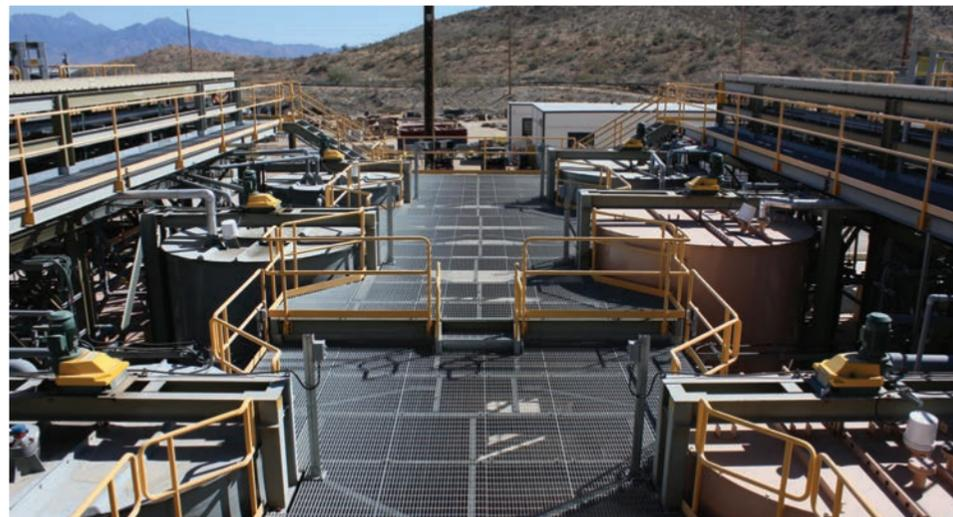
Columns house fluidized beds where the ion exchanges process takes place.
